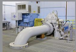
Open air and enclosed pump station units are designed to increase the pressure in the pipeline in order to maintain flow to keep the liquid petroleum moving at about walking speed.
